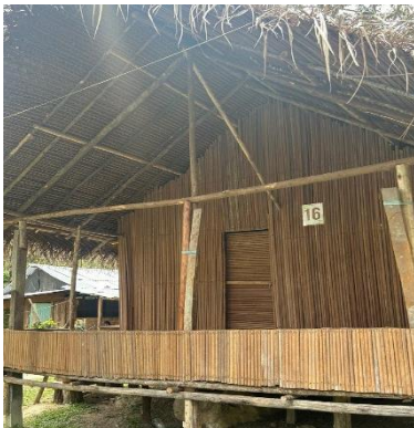
Figure 3: Chalet Gepeh (wall made from bamboo)
