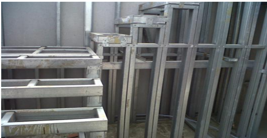
Plate 5.1.4 Showing The Staircase Carcass
