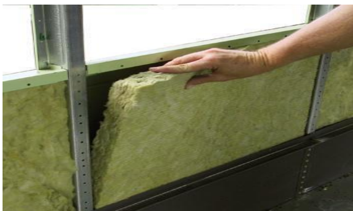
Plate 5.1.2 Showing the Mineral Wool Being Used as Insulation Within The Panels
