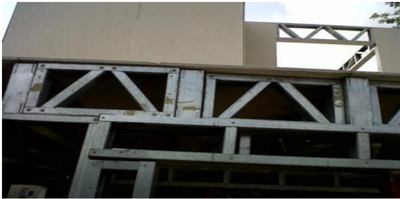
Plate 5.1.3 Showing The Lattice And The Kalsi Board Used For The Floor Slab
