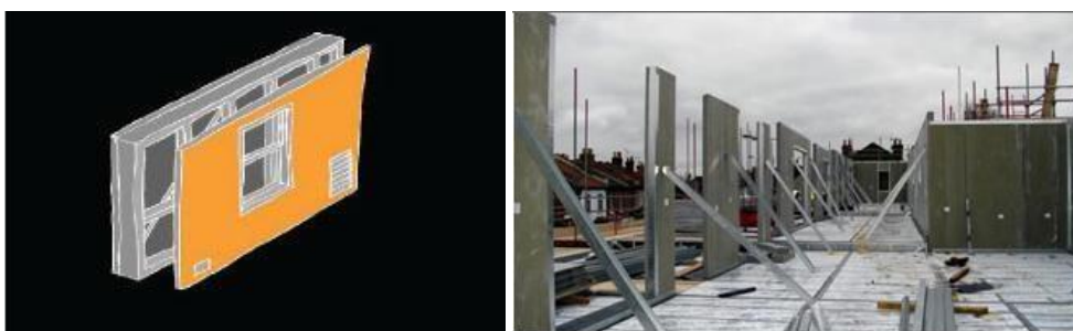
Figure 2 .0 Showing The Panelsystem Of Prefabrication
