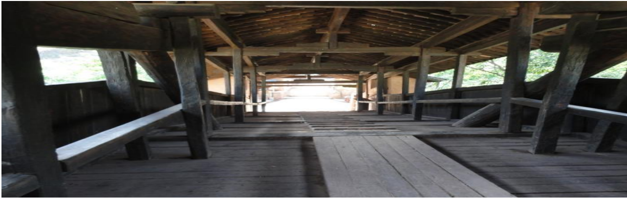
Fig. 6 Fengyu Ancient Bridge is a public semi-open space
