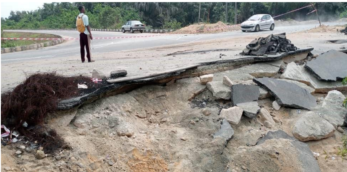
Plate 1: The eroded flexible pavement at the junction to the Cargo Airport along Amassoma Road ( 1 Adedokun, 2022)
