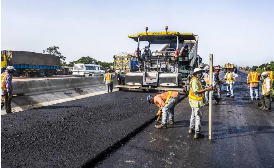
Fig 1 Lagos-Ibadan Expressway Expansion Project
