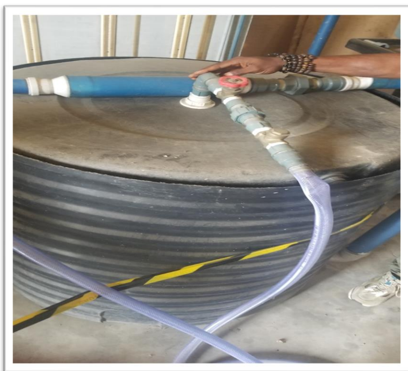
Fig.2.0 Lccal Biodigester( anaerobic) after consturctiom.
