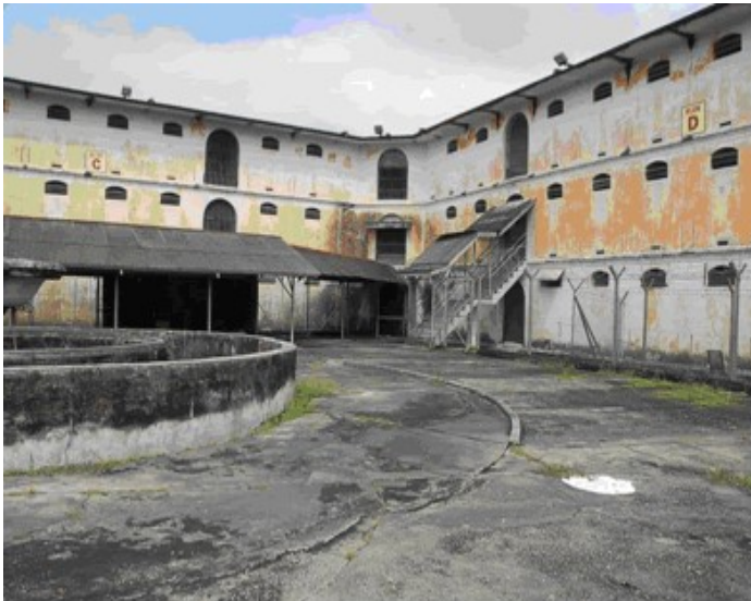
Figure 0.9: Back section of the abandoned Penjara Pudu.
