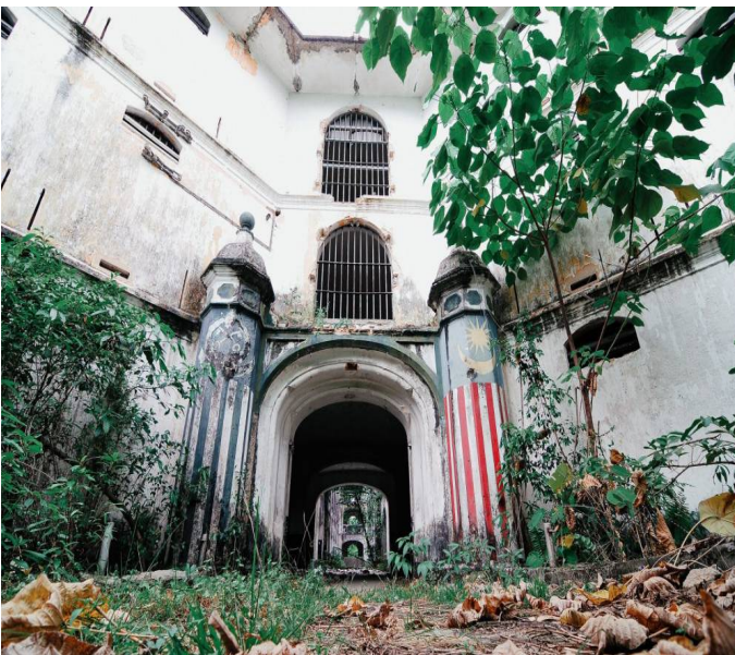
Figure 0.4: The sub main entrance of the abandoned Penjara Pudu.
