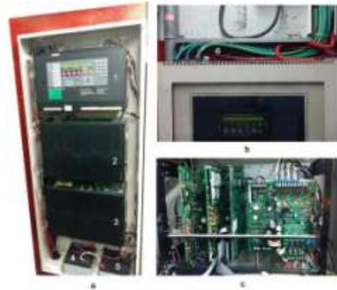
Fig. 4 Control panel (cabinet) of fire alarm (a) with three control units (1, 2 and 3) and accumulators (4, 5); 6 (b) - external multi-core cables, connected to internal electronic circuit of the cabinet; c - microelectronic "internals" of one of three control units of the cabinet.
