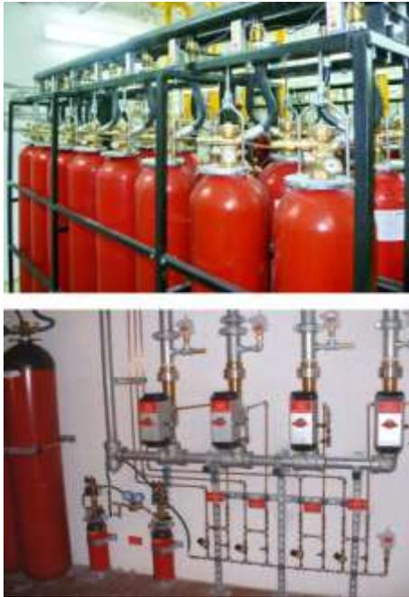
Fig. 2 Components of centralized gas fire suppression system
