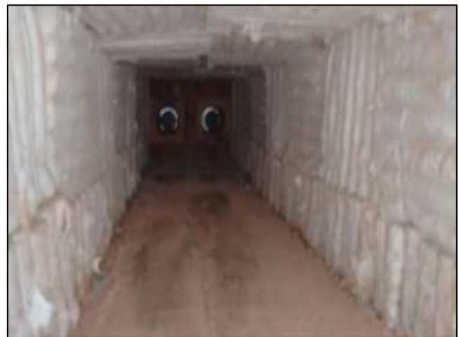
Fig-1 Inside view of the fire chamber with terrawool as insulating material
