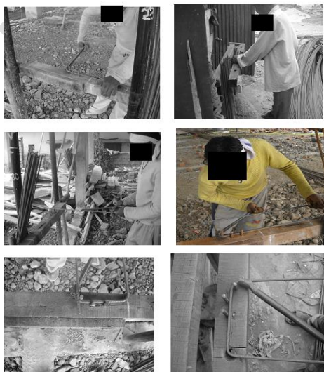
Figure 3 Traditional method of stirrup making
